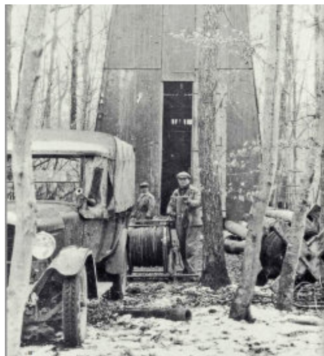
Logging survey at the Pechelbronn oil field (1928), Alsace, France. This is the same well in which Henri Doll, Roger Jost and Charles Scheibli, conducted the first electrical resistivity well logging operation in September, 1927. Source: Schlumberger.
